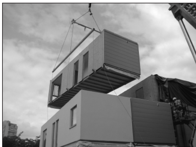
Figure 1. Partially open-sided module with load-bearing walls (courtesy PCKO Architects)
